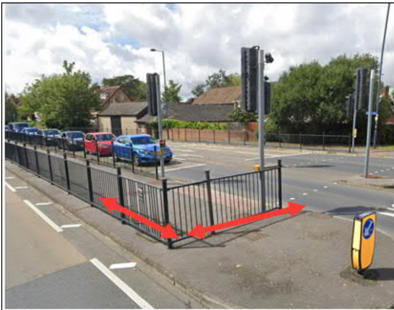
Figure 4: Existing pedestrian guard rail to be removed, set aside and reinstated.
